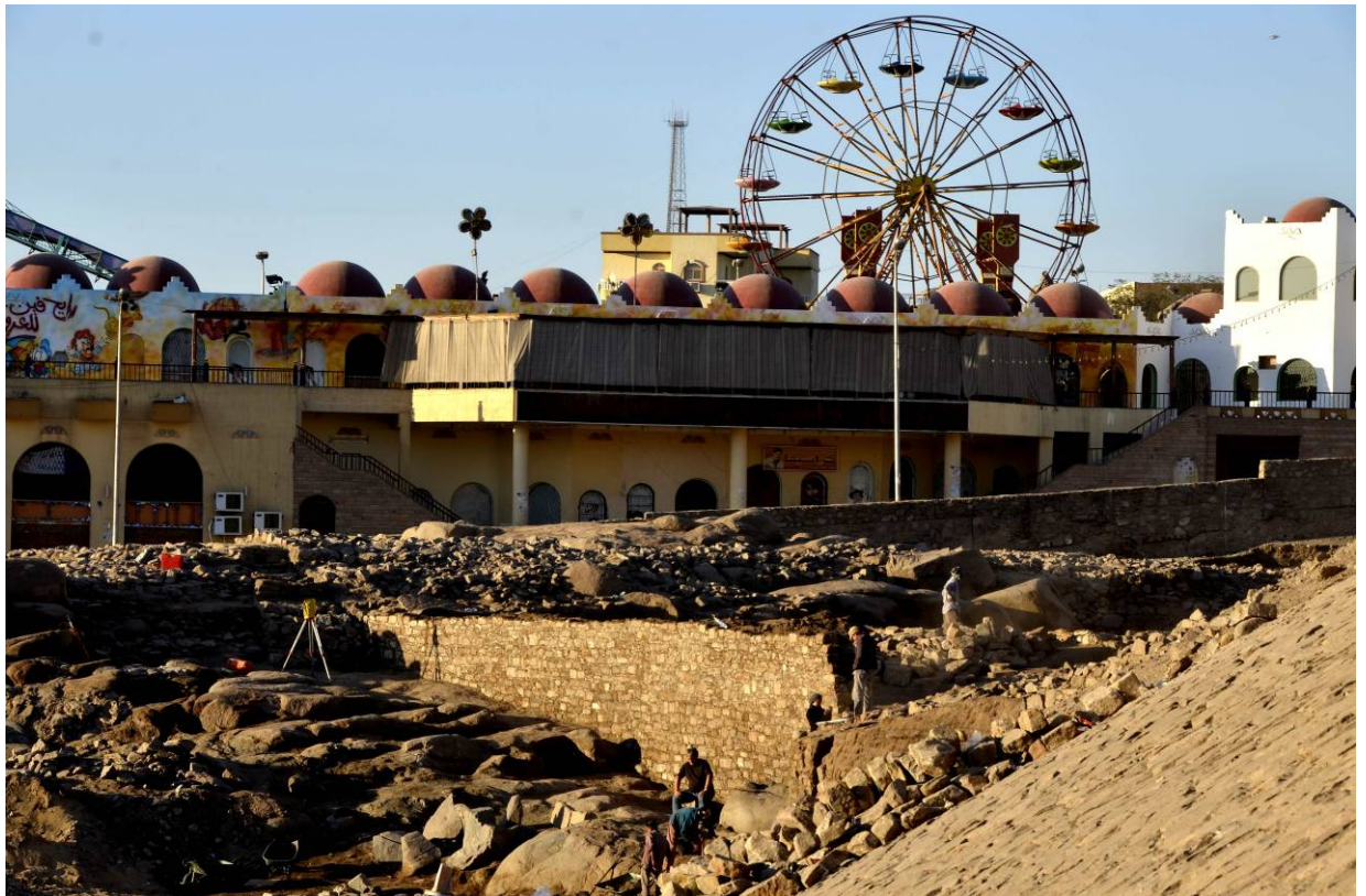
Fig. 2: Area 2: Conservation of the town-wall (photo: SIK/AK).
